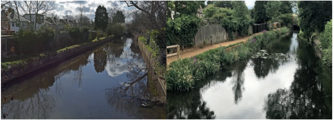
Duke of Northumberland River: canalised banks before restoration After installation of coir rolls & marginal planting
