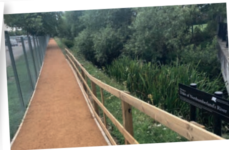
DNR after access improvement works
